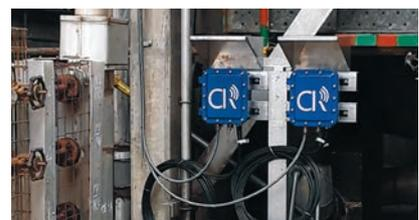
CR corrosion sensor mounted along a horizontal pipeline.
